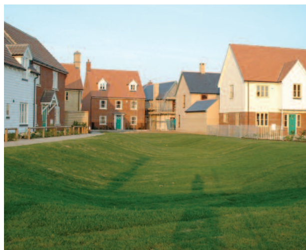
Infiltration basin in dry state, Ipswich
