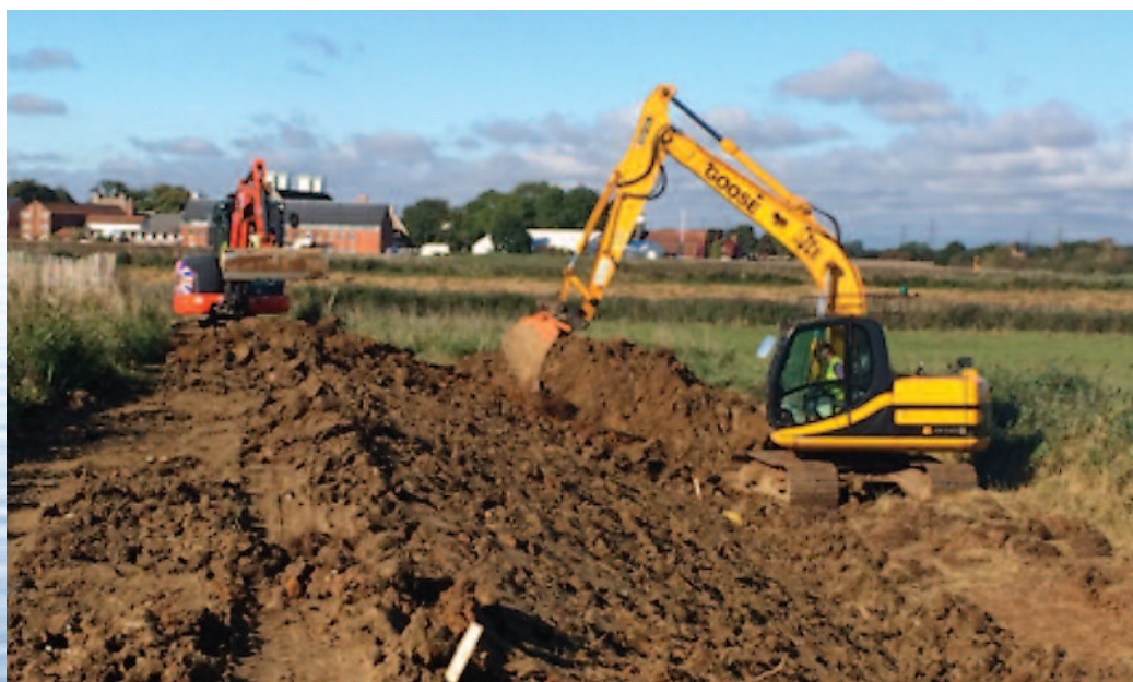
Repairs to flood bank
