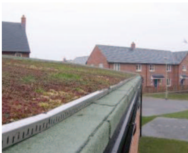
Green roof on a shed
